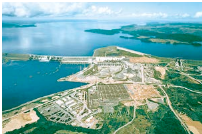
Hydroelectric power station Tucuruí, Brazil: 23 x 390 MVA, 11 THYRIPOL static excitation system from Siemens
