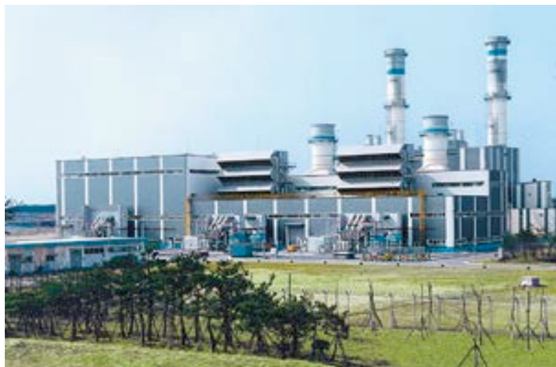
Gas and steam turbine power station Bugok, South Korea: 2 x 205 MVA, 1 x 207 MVA, 3 THYRIPOL static excitation systems from Siemens
