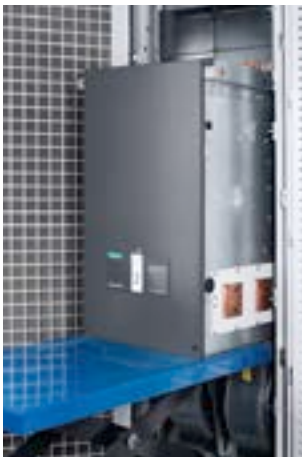
Replacing the converter module while the system is operational
