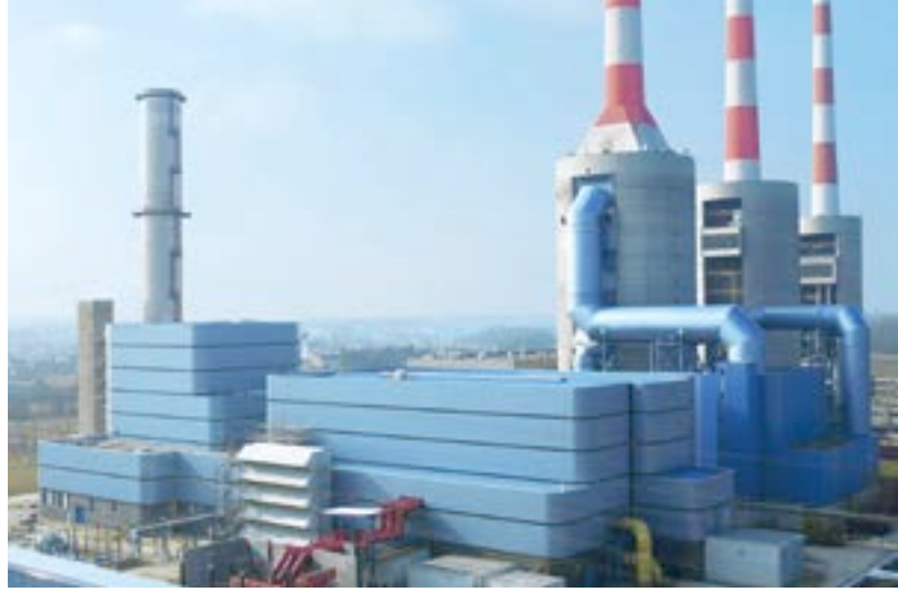
Gas and steam turbine power station Irsching Block 4, Germany: 561 MW, THYRIPOL static excitation system from Siemens
